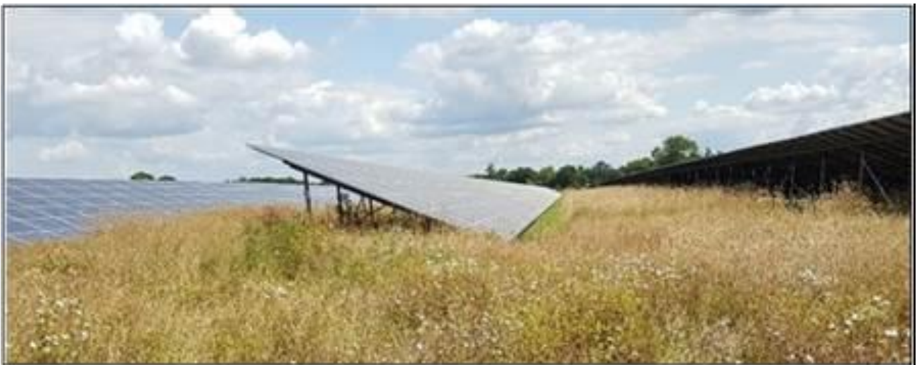
Plate 1: Site where a “Shade Cut” has been employed during the growing season to prevent shading of panels but allow flowering meadows elsewhere.
